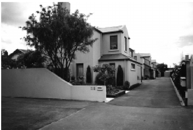
Living 2 zone housing development
