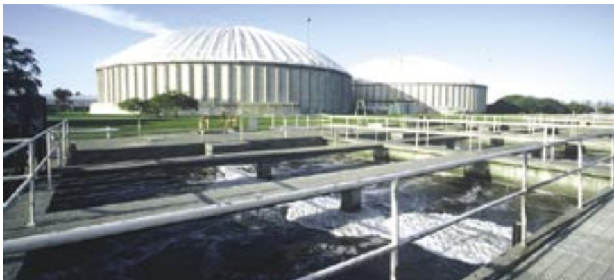
The oxidation tanks at the Wastewater Treatment Plant, in Bromley
