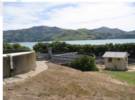
Akaroa Wastewater Treatment Plant
