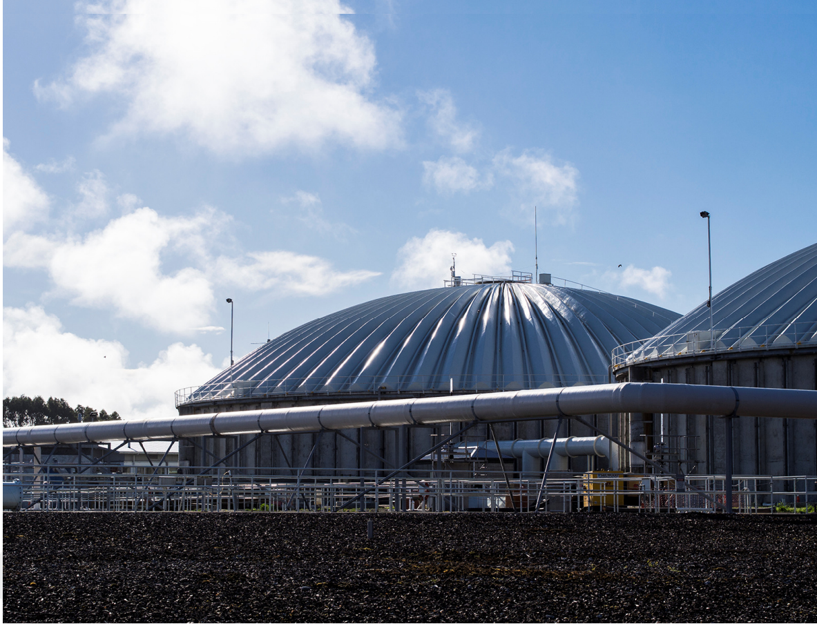
Christchurch Wastewater Treatment Plant
