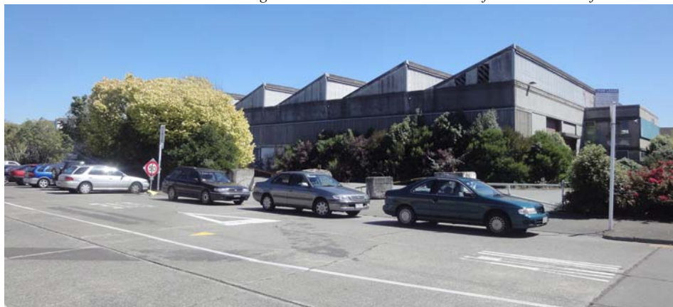
Below: The vacant Rail Shed B building with its distinctive saw-tooth roof on the corner of Cass and Colombo streets
