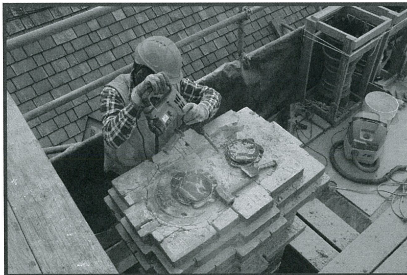
Neil Boxall deconstructing chimneys damaged by the 22 February Earthquake
