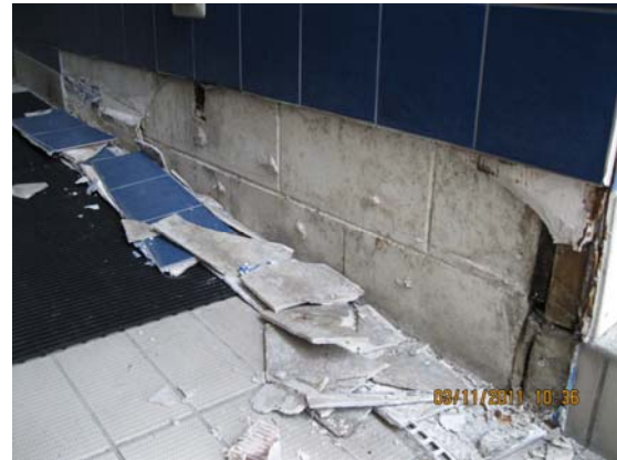
Cracked and delaminated tiles below mezzanine level (a result of differential settlement).
