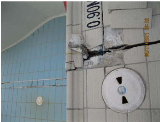
Cracked and deformed pool edge at Leisure pool, levels have dropped across crack extent (typical).
