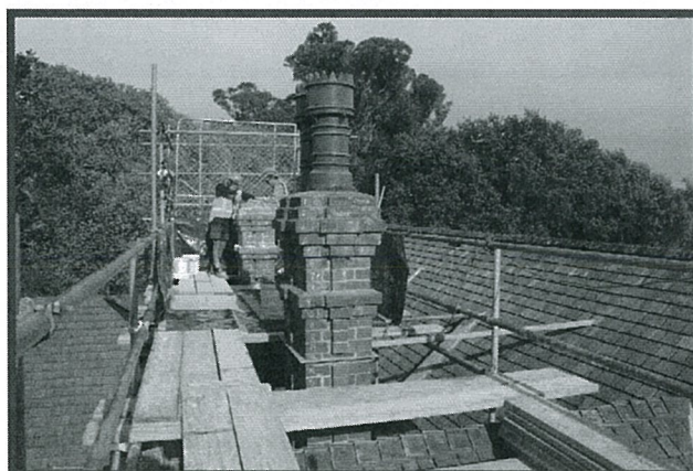
Chimney deconstruction following the 4 September 2010 earthquake
