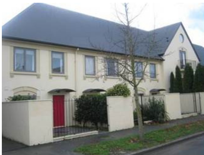
Photo 1: Chester Street East
