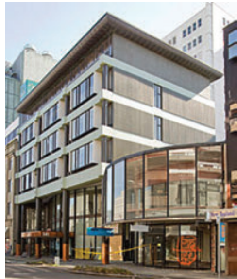
2: Building before Demolition
