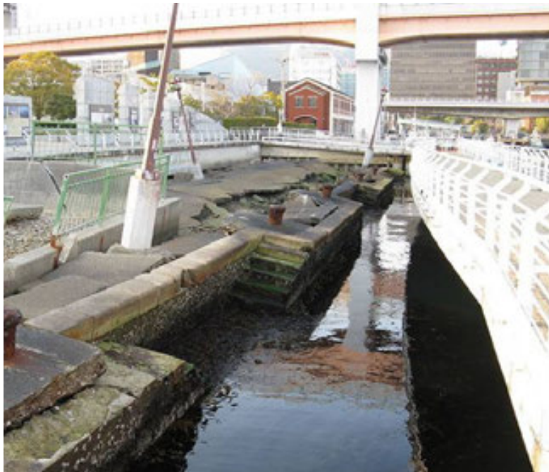
Damaged landscape from the Great Hanshin Earthquake in Kobe, Japan, 1995, is preserved as a memorial.
