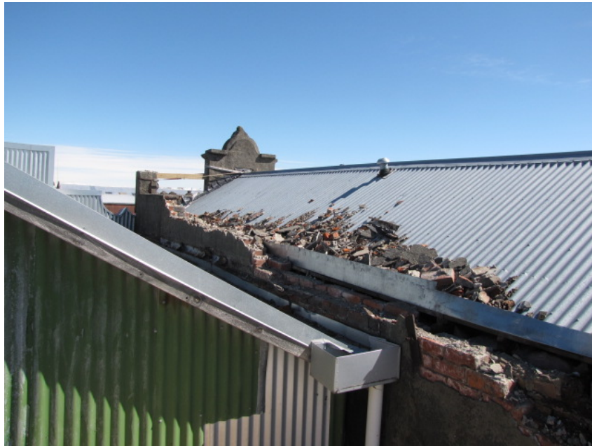
Figure 3: damaged firewall
