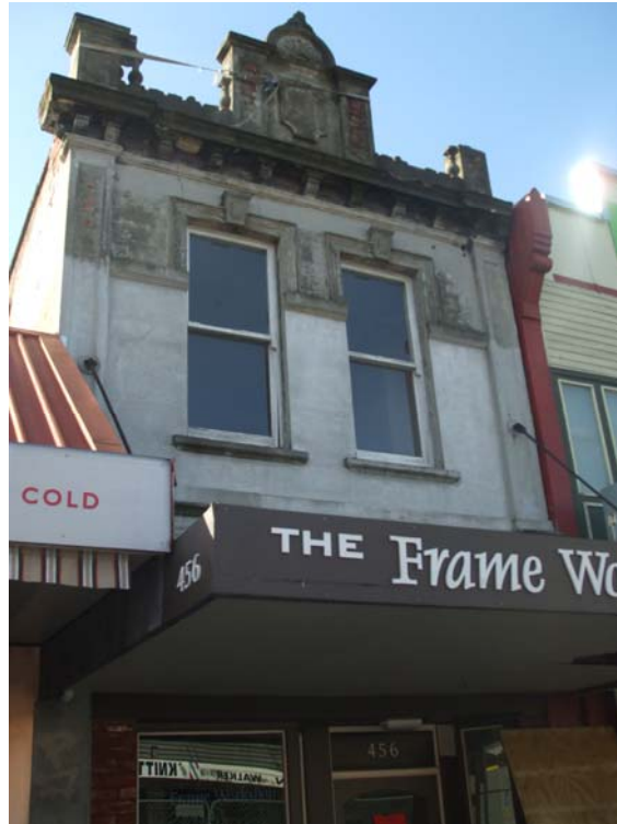
PHOTOGRAPH: 456 COLOMBO STREET
