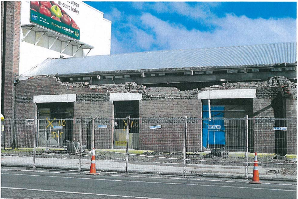
North Wall single storey section
