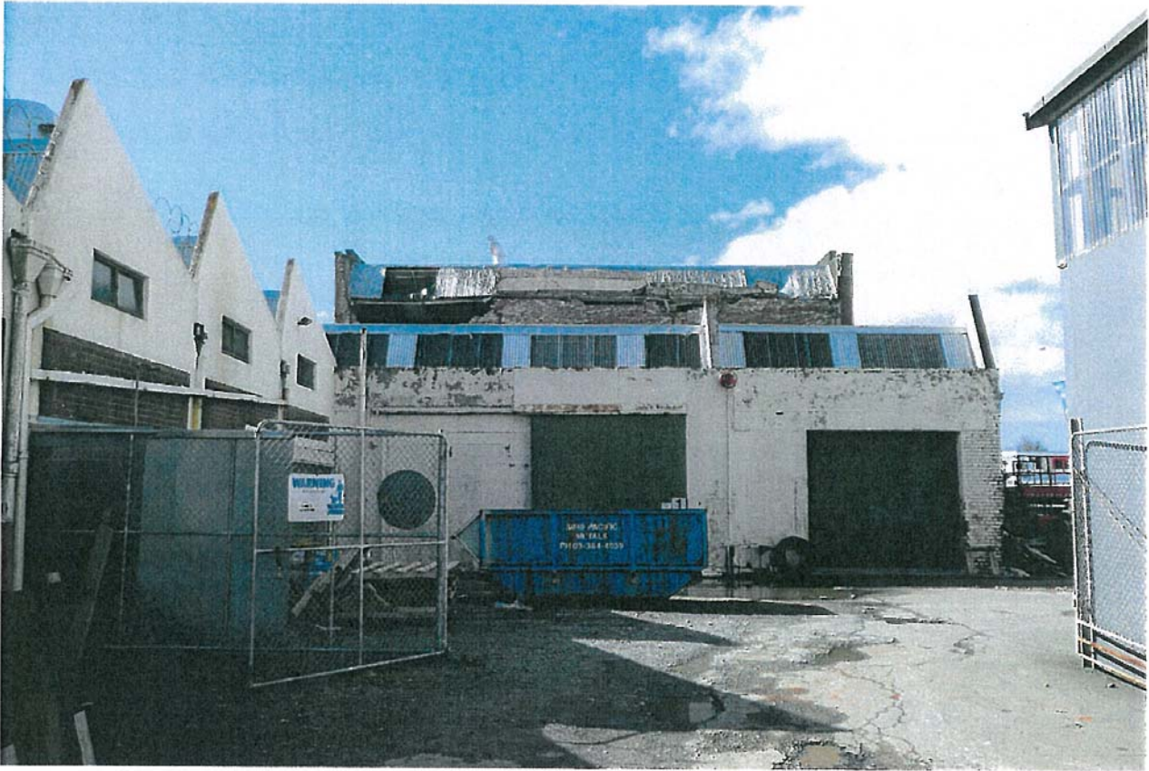
South Wall Two Storey building
