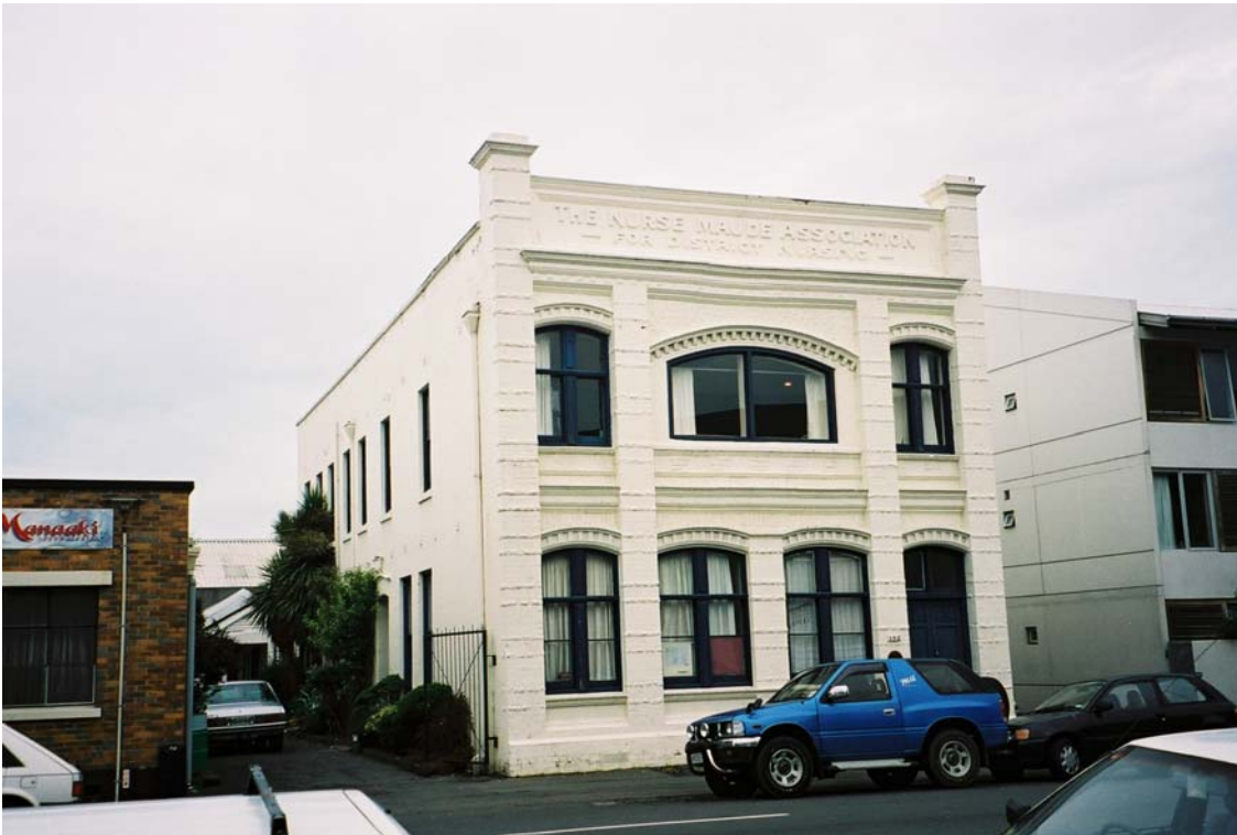
PHOTOGRAPH: 192 MADRAS STREET
