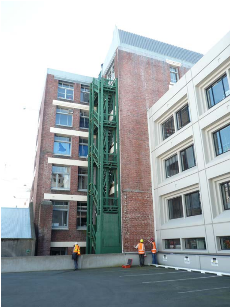
Rear of property, east façade
