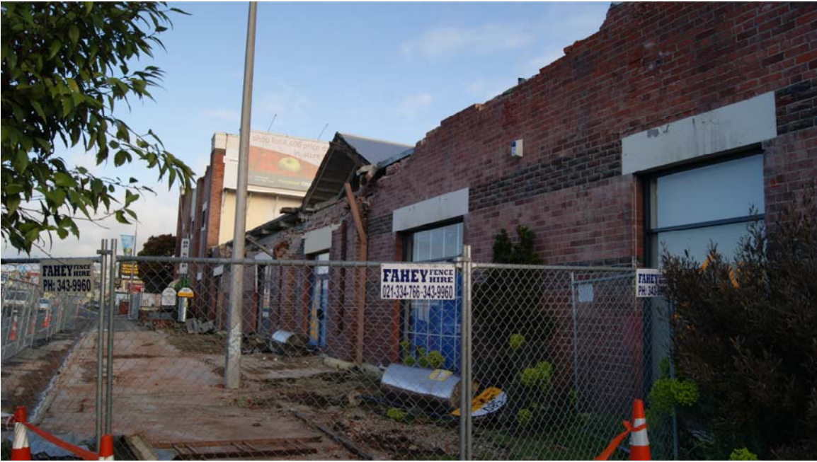
North Wall single storey section
