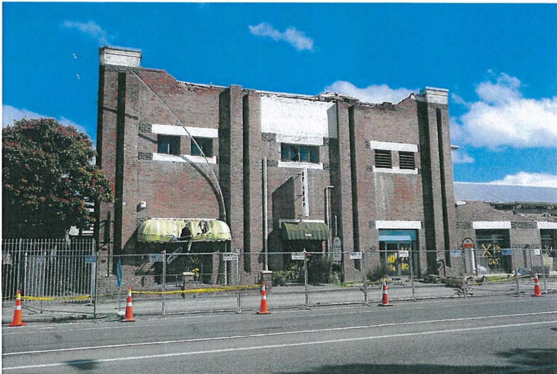
North Wall two storey Building
