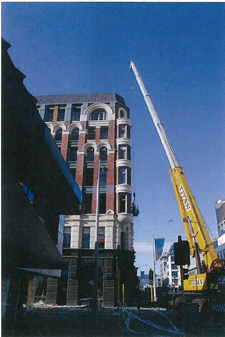
Image 4. Crane positioned in intersection.
