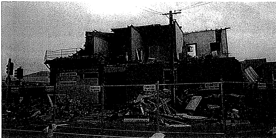
Figure 1: View from north
