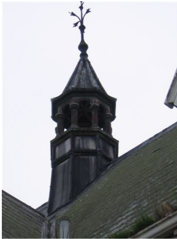
The ventilation fleche which surmounts the building. (Photo: J May, 2005 for Conservation Plan, 2006)
