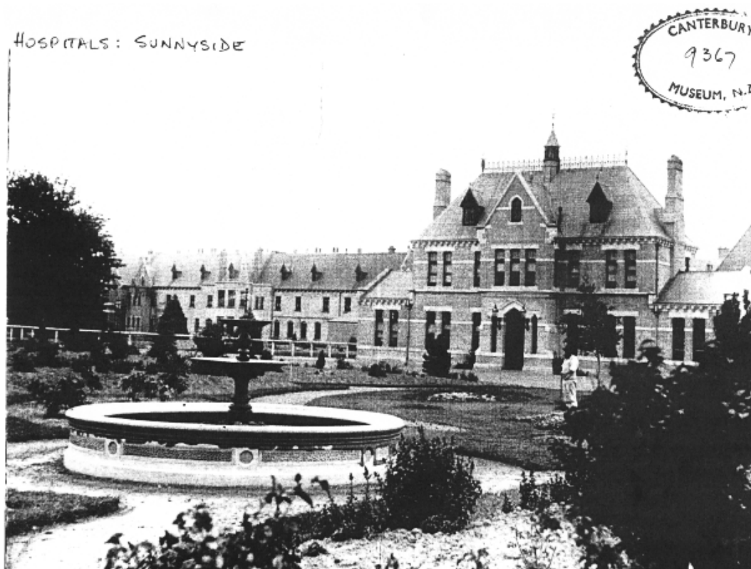
The Administration Building c.1895? The photo includes the fountain and formal garden beds in front of the building and behind it, part of the earlier hospital complex designed by Mountfort. (Photo: Canterbury Museum, No. 9367, copied from Christchurch City Council files.)
