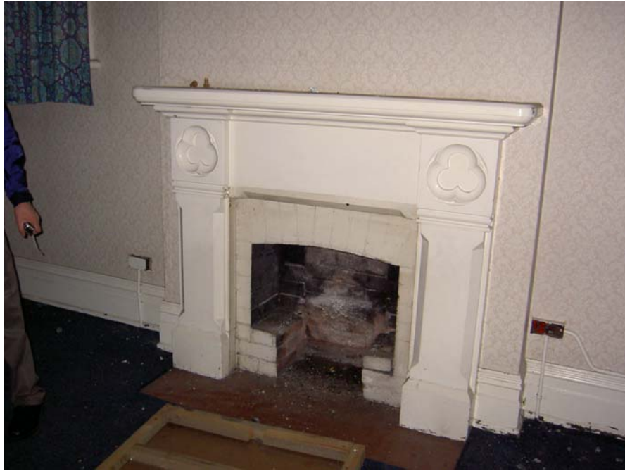
One of the remaining fireplaces. The skirtings are original. (Photo: J May, 2005 for Conservation Plan, 2006)
