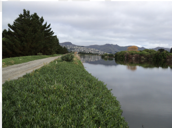
Oxidation pond at Bromley
