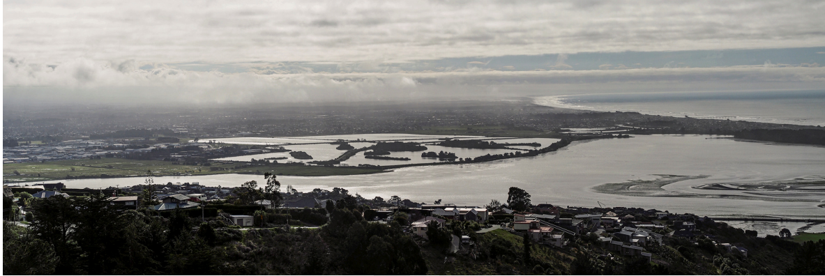
Oxidation pond at Bromley
