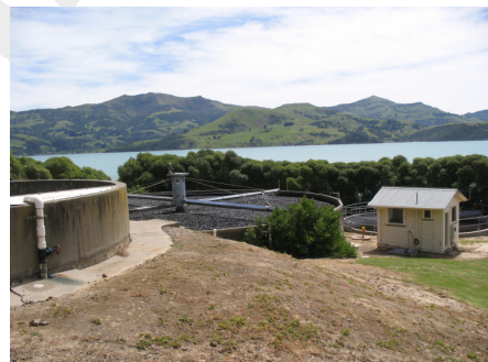
Akaroa Wastewater Treatment Plant
