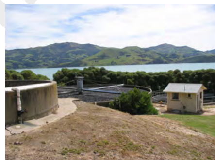
Akaroa Wastewater Treatment Plant
