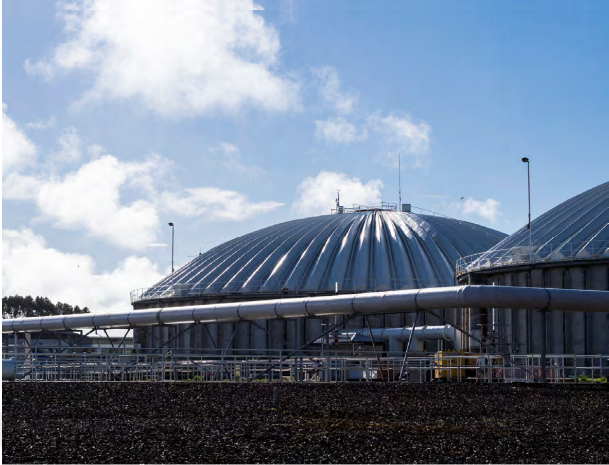
Christchurch Wastewater Treatment Plant
