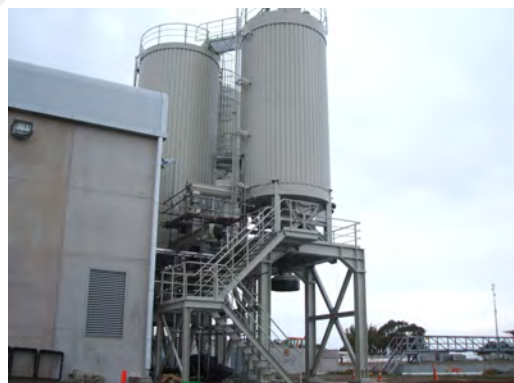
Biosolids Drying Facility at Bromley
