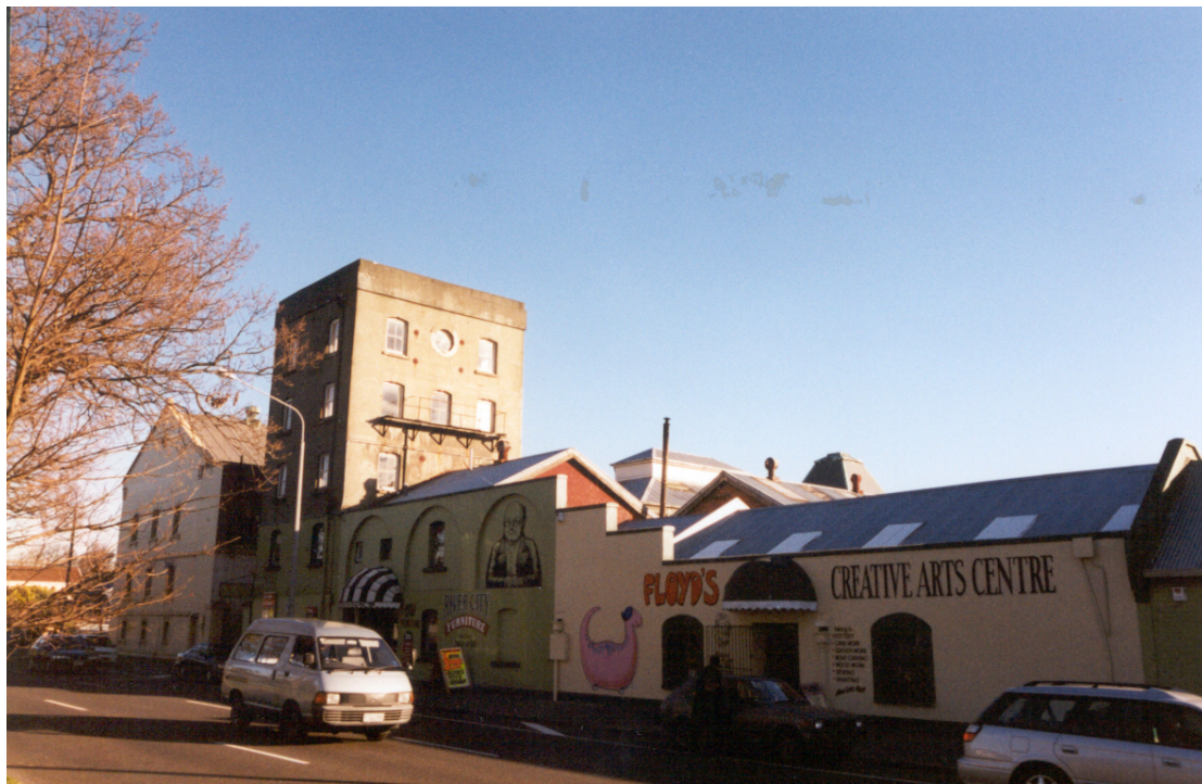
WARD'S BREWERY COMPLEX, FITZGERALD AVENUE PHOTOGRAPH: 2010 PRIOR TO CHRISTCHURCH EARTHQUAKES
