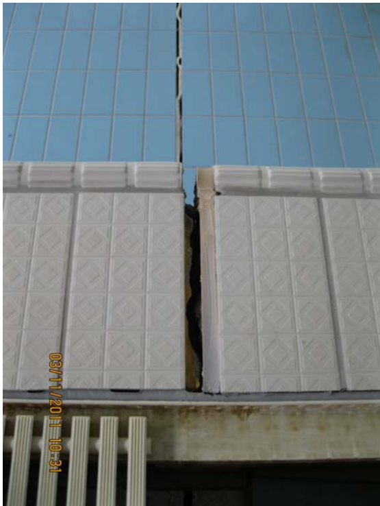
Open Movement joint with longitudinal movement visible (typical).
