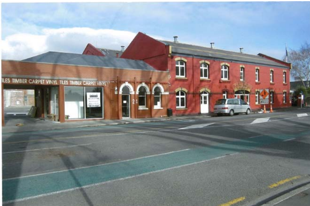
Kilmore Street frontage
