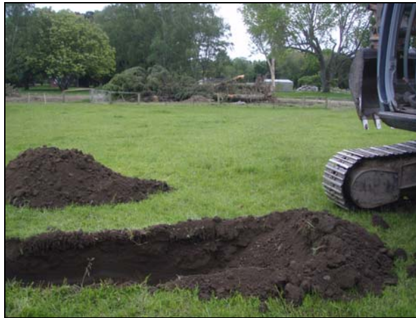
Photograph 1: Excavation within the suspected landfill
