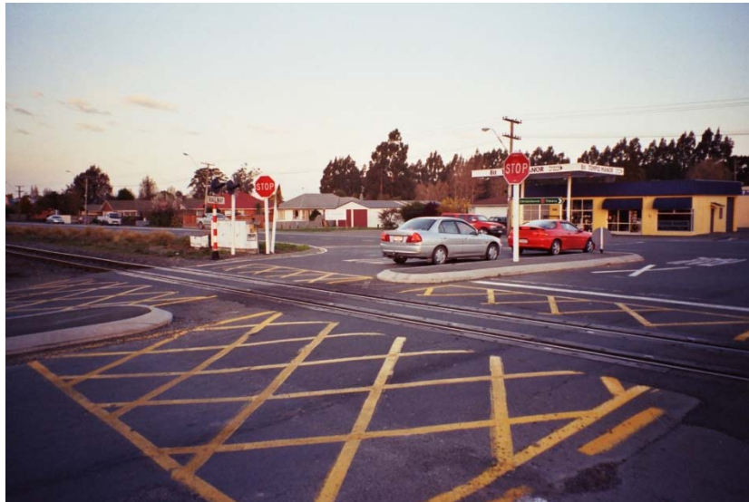
Photograph 1: Kirk Road / SH1 Intersection and level crossing
