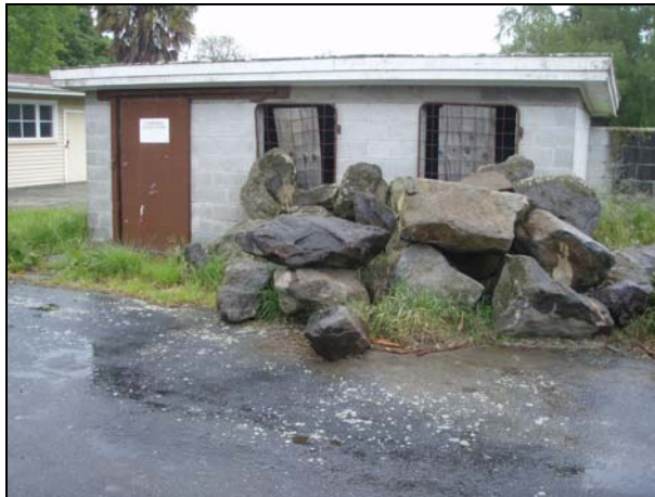
Photograph 5: View of the former flammable shed in the northern portion of the site
