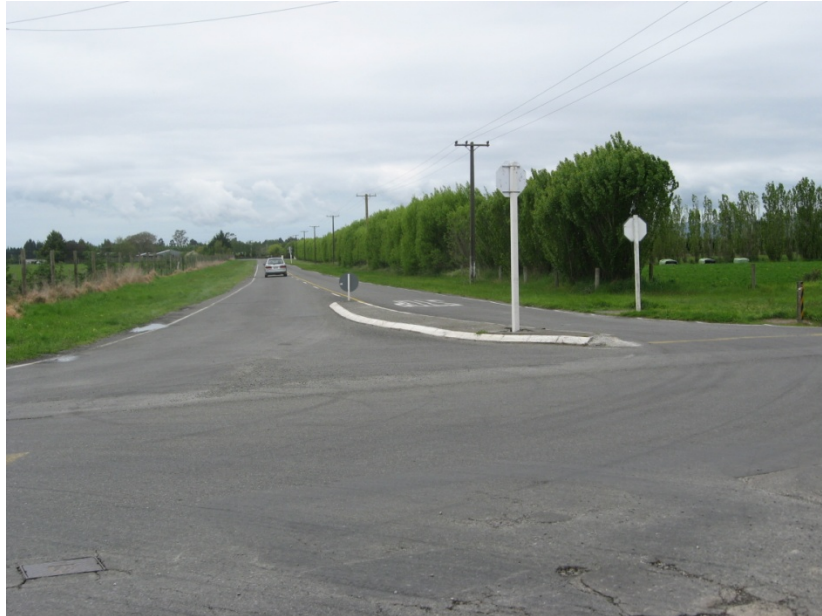
Photograph 3: Maddisons Road at Maddisons Road / Kirk Road intersection
