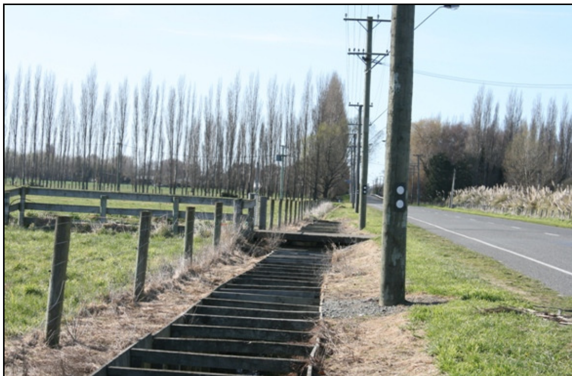
Photo 5 – Prestons Road looking east towards Mills Road
