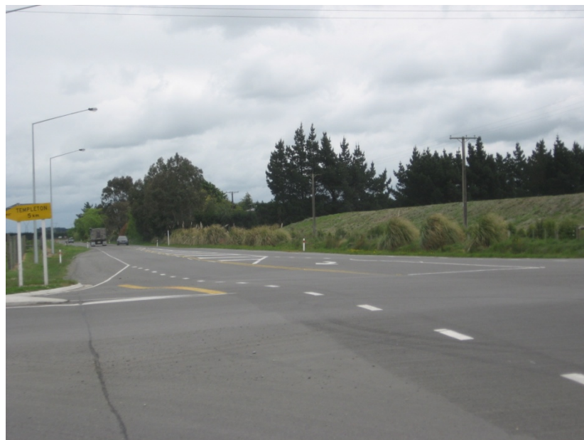
Photograph 4: SH73 / Kirk Road intersection
