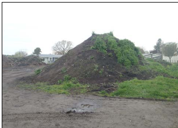
Photograph 6: View of the new stockpiles towards the western site boundary
