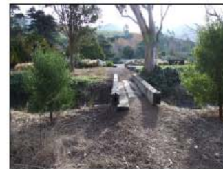
G EXISTING WOODEN FOOTBRIDGE BETWEEN THE DOMAIN AND REST AREA
