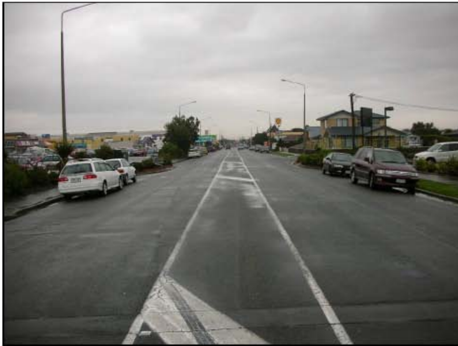
Figure 2: Typical Hawke Street Cross Section (Looking westward directly outside the 'Woolworths' access)
