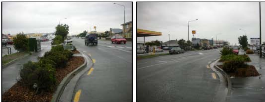
Figure 3: Hawke Street Kerb Extensions (Left: Kerb extension outside Keppel Street; Right: Kerb extension outside Howe Street)
