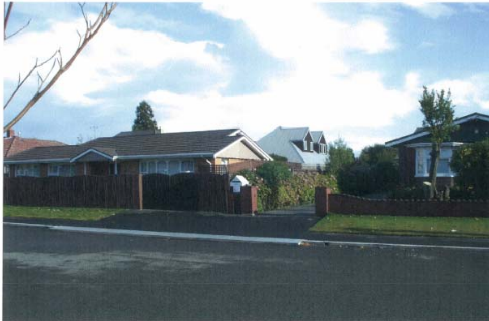
Photo 1- Excessive crossfall on the western side of Chilcombe St
