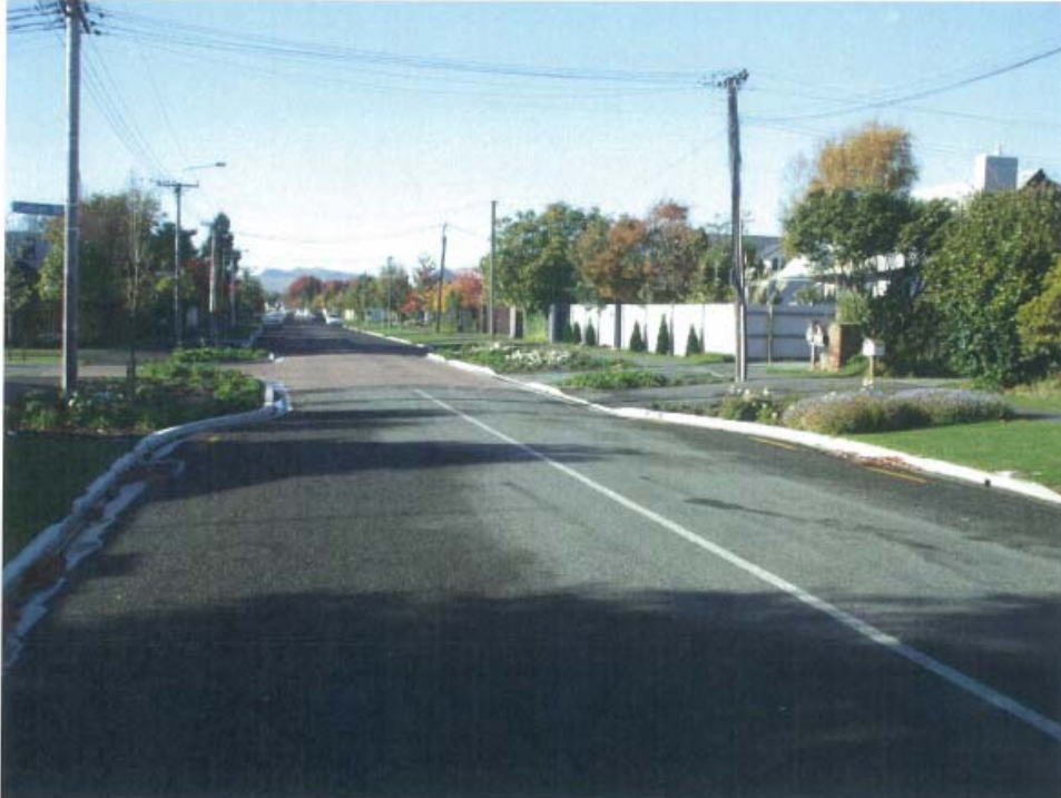
Photo 4 - Threshold treatment at the Lothian St and Hamilton Ave intersection
