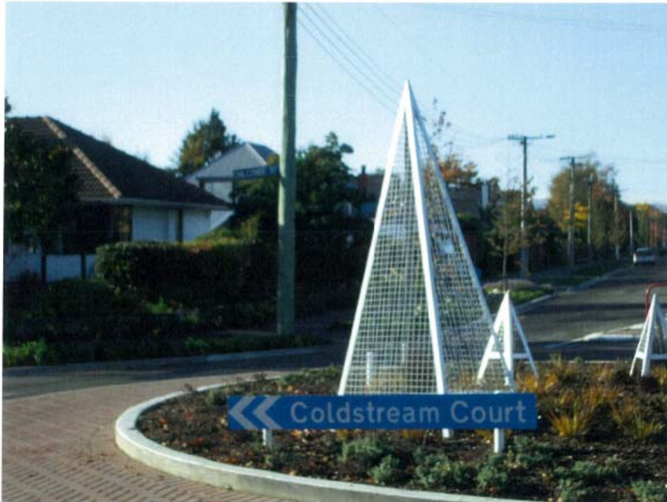
Photo 2 - Incorrect direction of street name sign
