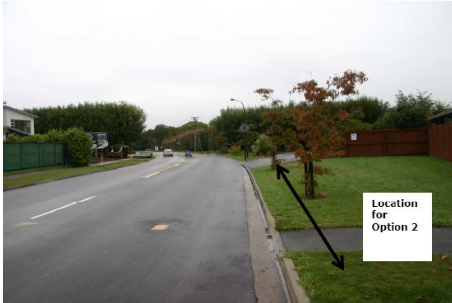
Hussey Road – Outbound stop opposite Styx Mill Country Club - Proposed bus stop location for Option 2
