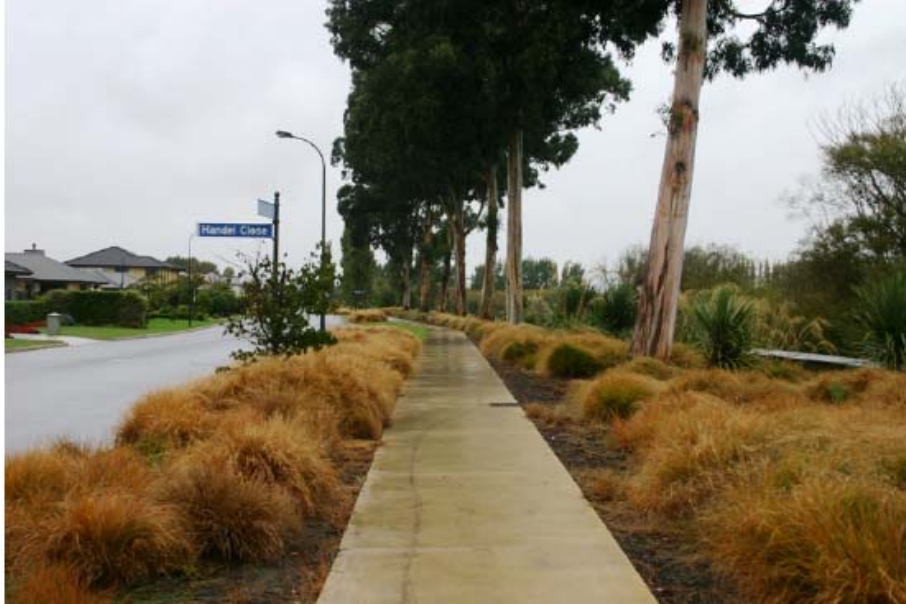
Saracen Ave – link footpath on south side of road
