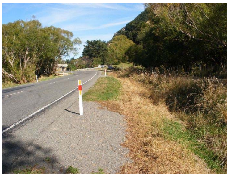
Figure 2 SH crossing point visible in background
