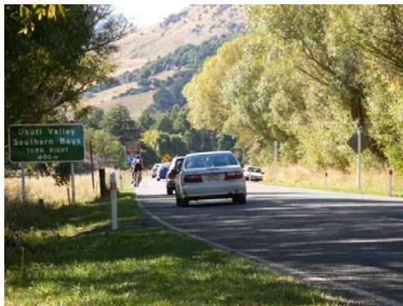
Figure 5 Lack of road shoulder north of existing crossing point
