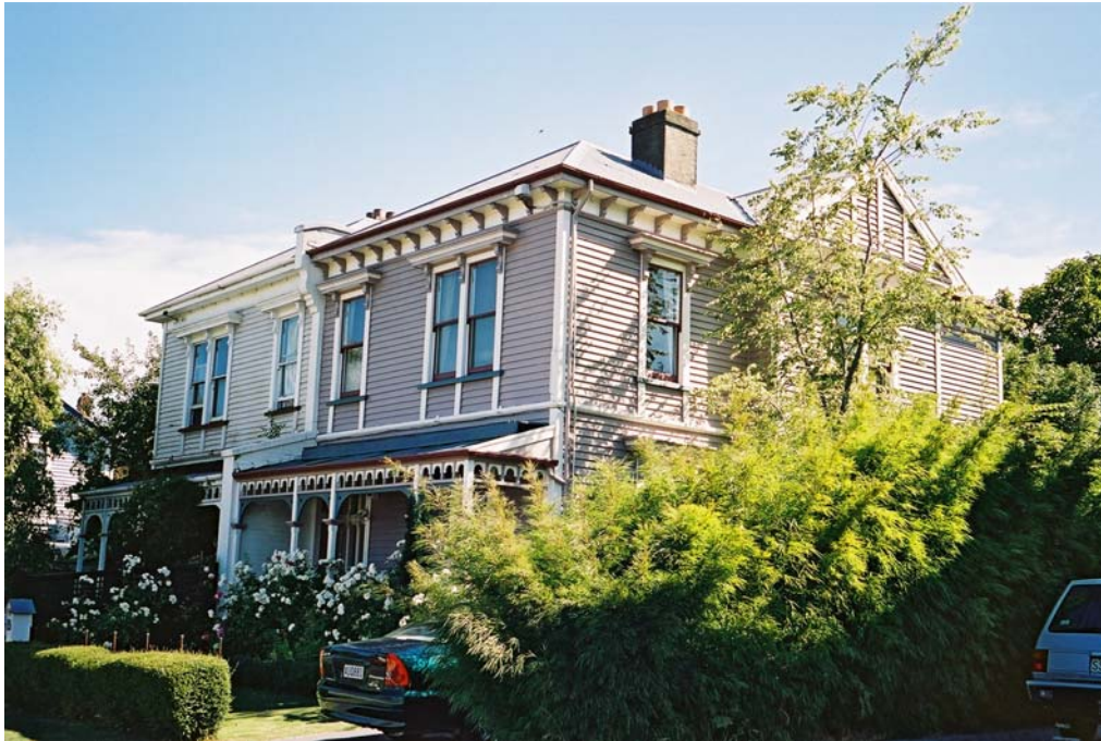
PHOTOGRAPH C2003 – 11 AND 13 CHURCHILL STREET
