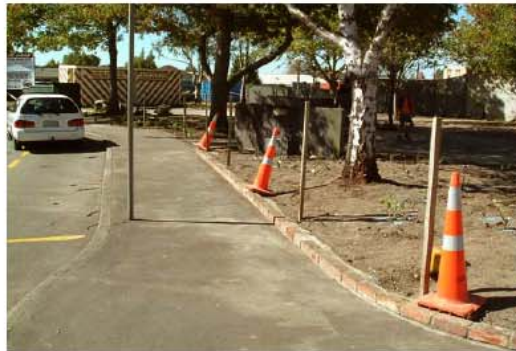
Photograph 9 – Planting Day The raised brick edge around the Rose Bed
