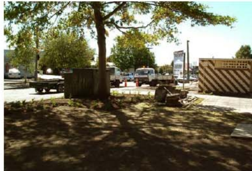
Photograph 13 – Planting Day View of the Orion Box and the side of the toilets
