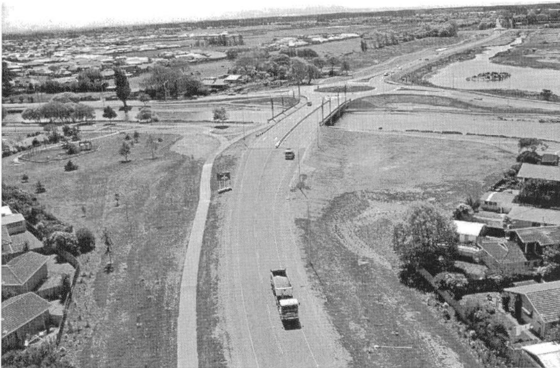
View of the recently opened stage of the expressway (looking from the south towards New Brighton Road)
