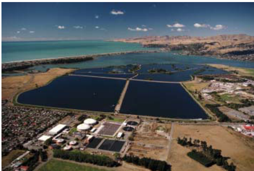
An aerial view of the Waste Water Treatment Plant.
