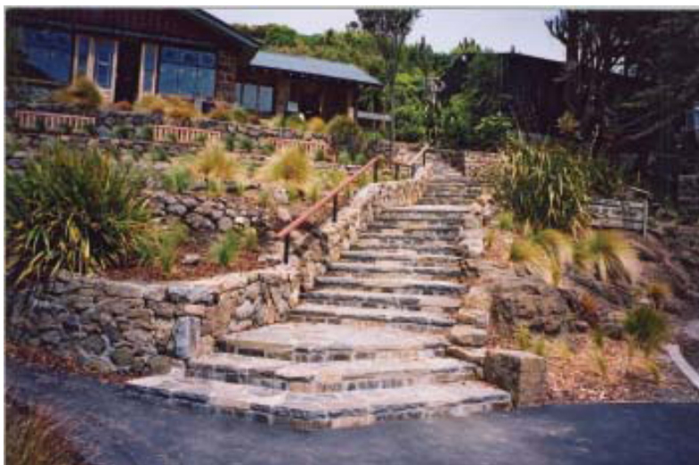
Recently reconstructed steps at the Sign of the Kiwi.
