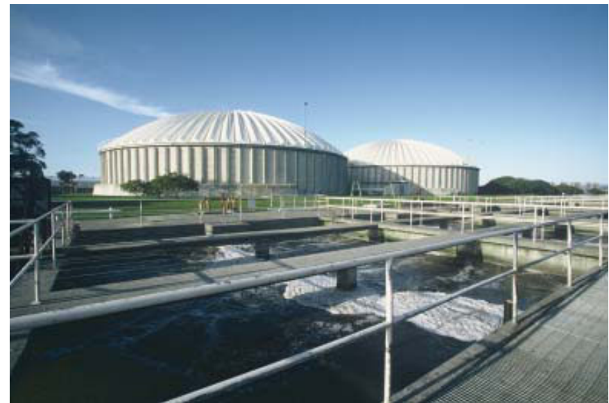
The Waste Water Treatment Plant.
