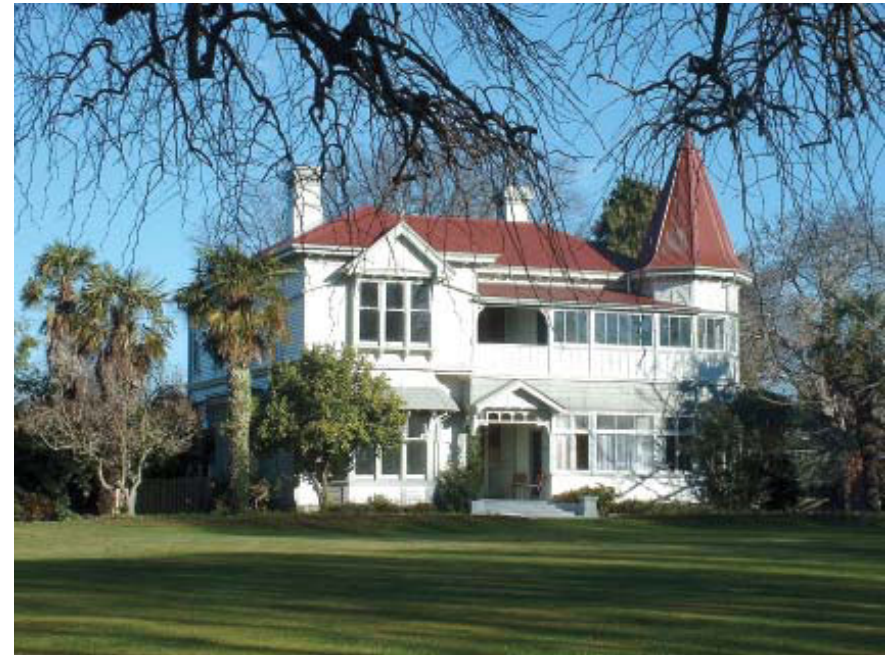
Avebury House- a recently developed community centre.
