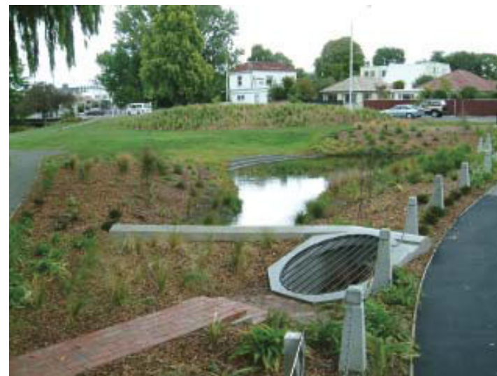
The recently developed Cambridge Green on the corner of Salisbury and Barbadoes Streets.
