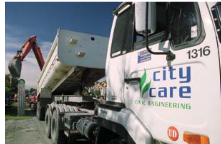
City Care replaces a water sub main.
