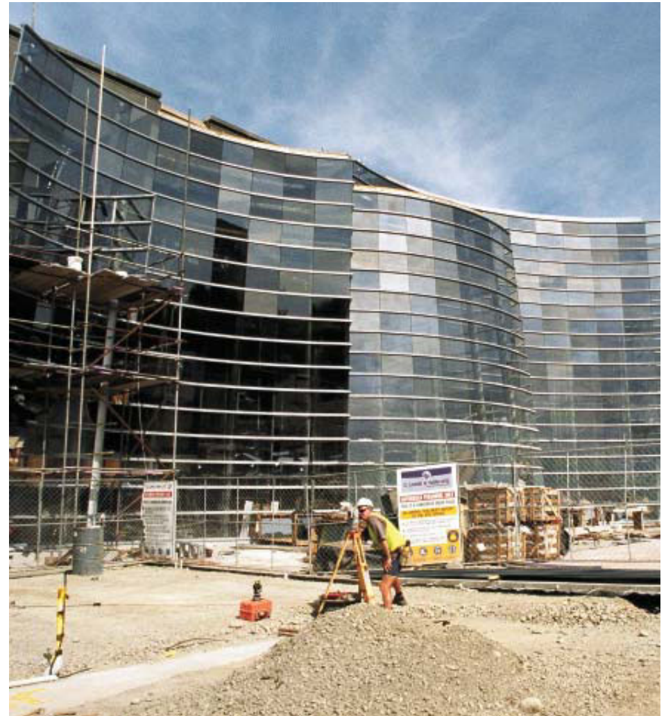
Construction work on the new Christchurch Art Gallery.
