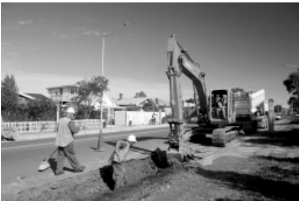
Kerb and channel work being undertaken in Woodham Road
