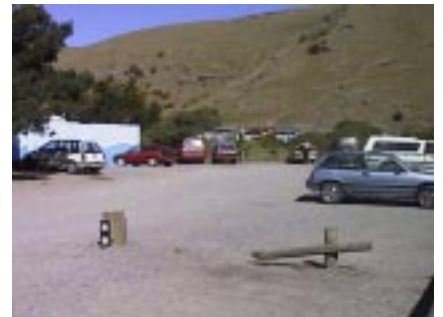
2 Broken posts and rails
