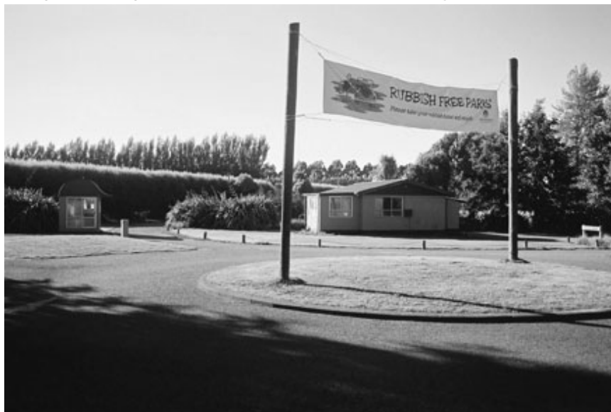
Figure 5 Existing Park Ranger's office / visitors centre at The Groynes entrance
