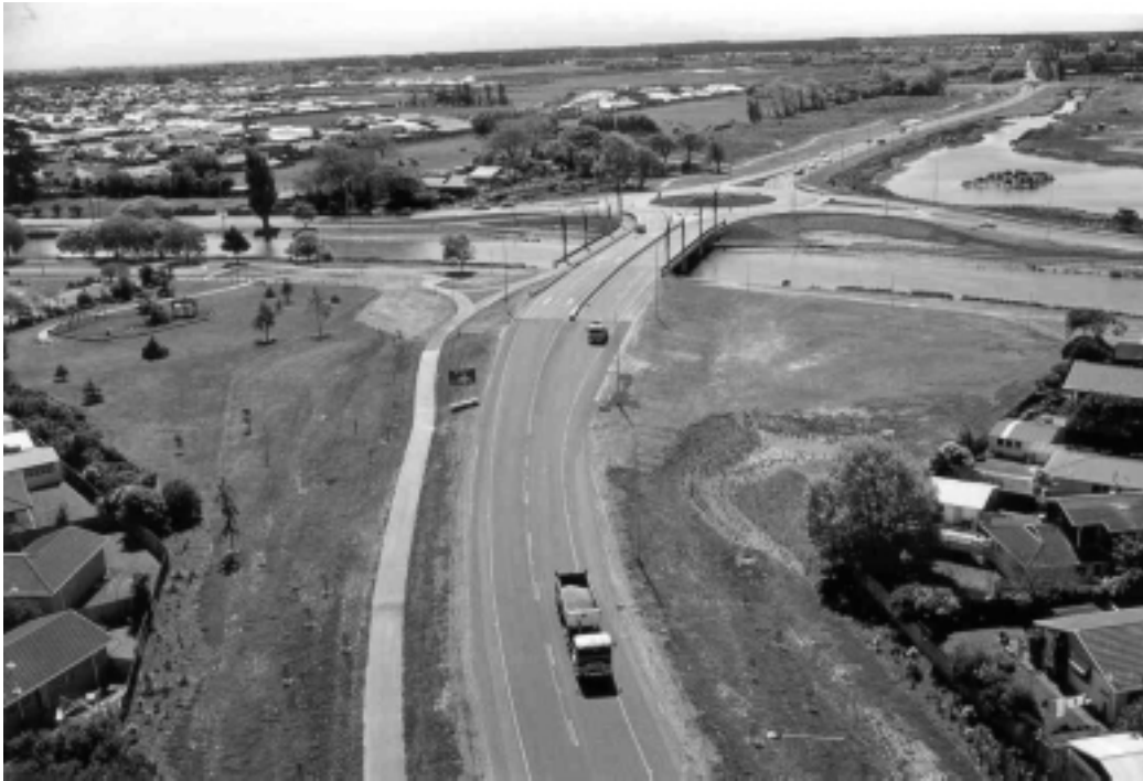
VIEW OF THE EXPRESSWAY AND RESERVE AREAS FROM THE SOUTH
