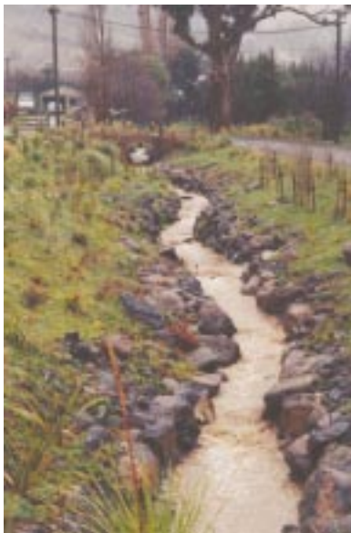
Erosion control work which has been completed by the Water Services Unit on the Butts Valley Stream.
