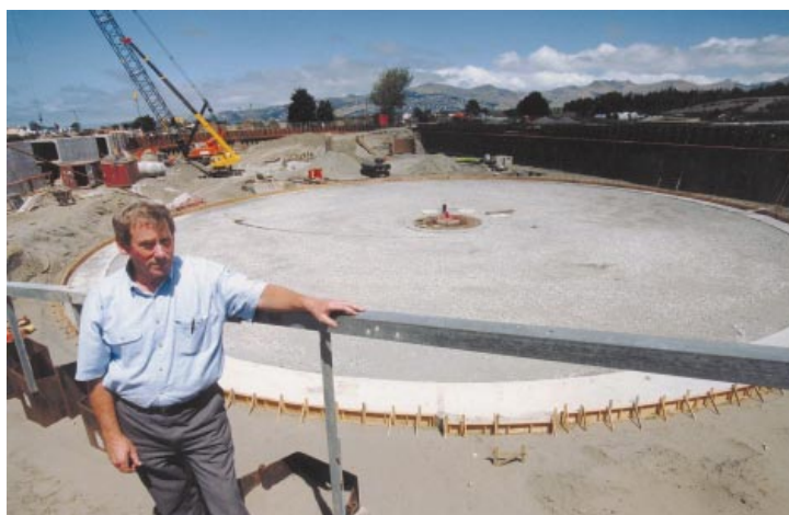
A view of construction work on one of the four new secondary clarifiers. This is part of the treatment Plant upgrade.
