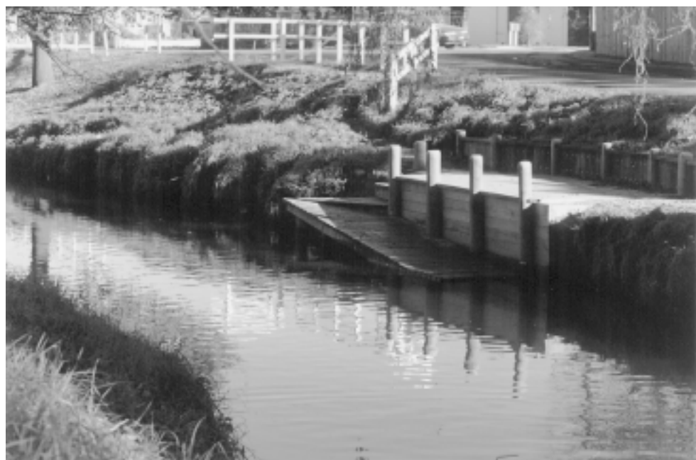
The Waltham Bridge River Jetty on Fifiel Terrace
