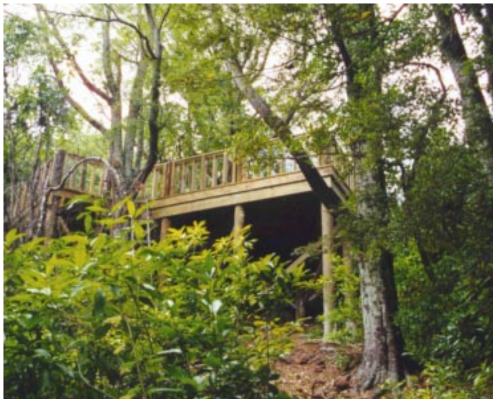
Looking up at one of the platforms of the newly completed Tawhairaunui Trail in Victoria Park. The new track gives people in wheelchairs or pushchairs easy access to the bush and views of the Port Hills
