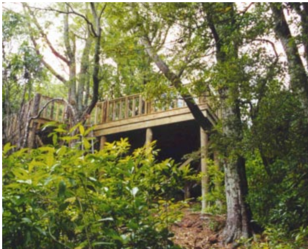
Looking up at one of the platforms of the newly completed Tawhairaunui Trail in Victoria Park. The new track gives people in wheelchairs or pushchairs easy access to the bush and views of the Port Hills
