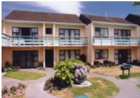
Manse Place 325 Main North Road, Redwood
