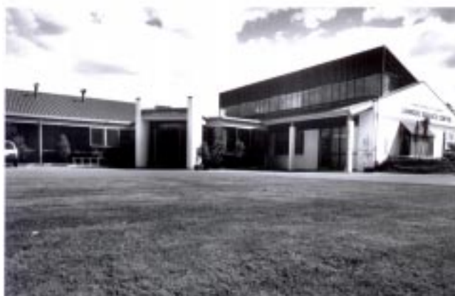
Linwood Service Centre
