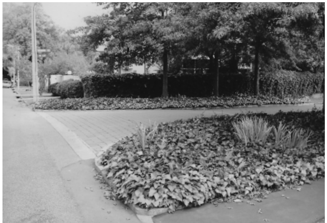
An example of threshold treatment and street landscaping
