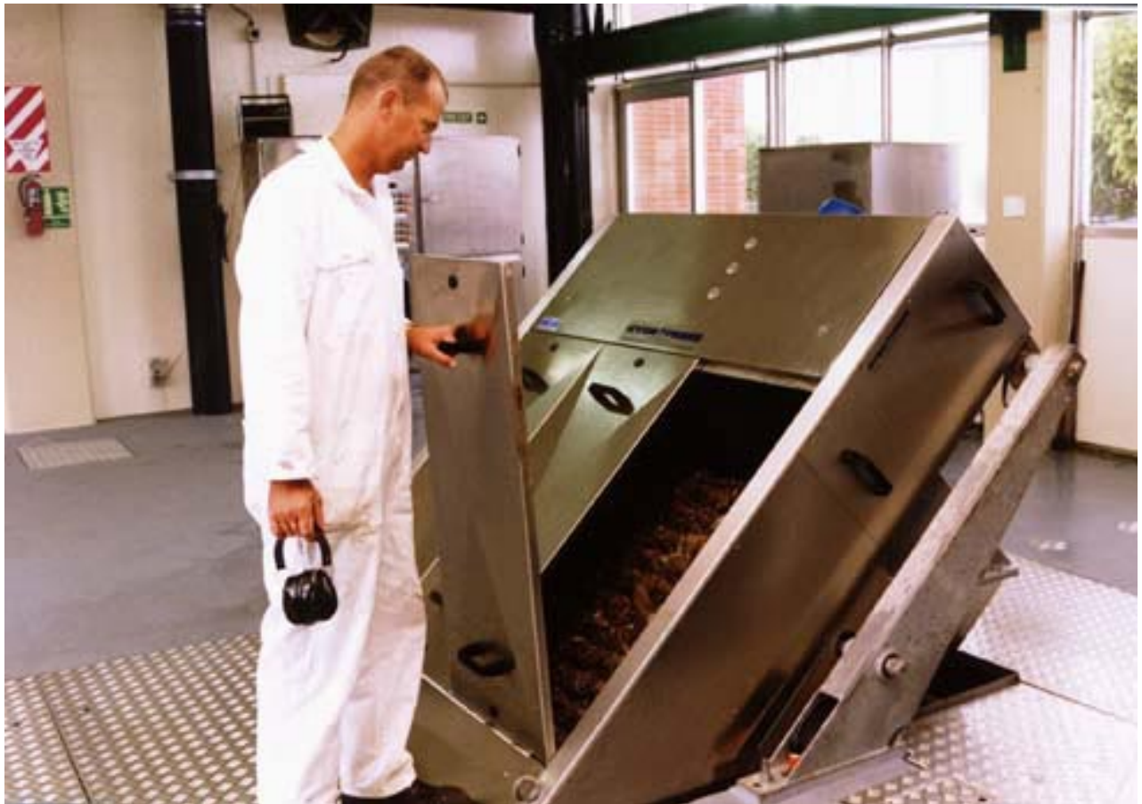
One of a series of new step screens installed at the city's wastewater treatment plant to filter out solid material. These screens are the first part of a $30 million plant expansion which will provide capacity for city growth for another 30 years.
