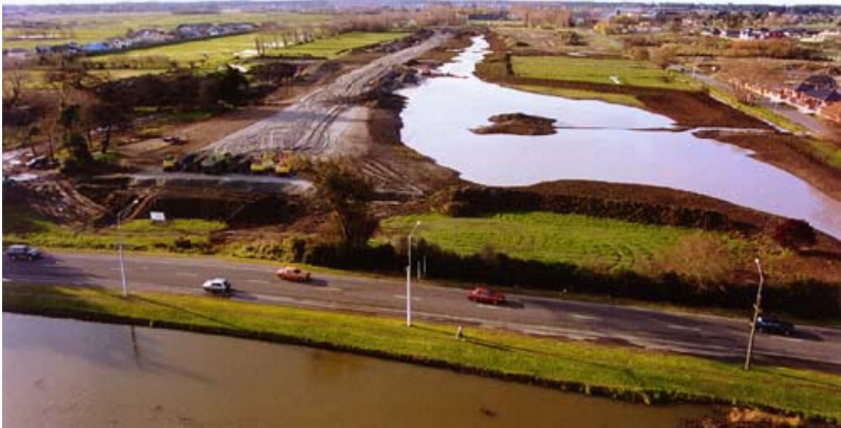
Woolston/Burwood Expressway construction and associated wetland development with New Brighton Road and the Avon River in foreground.
