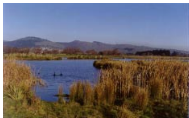
Wigram wet pond and stormwater retention basin.
