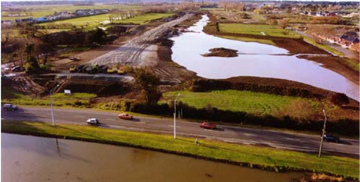
Woolston/Burwood Expressway construction and associated wetland development with New Brighton Road and the Avon River in foreground.
