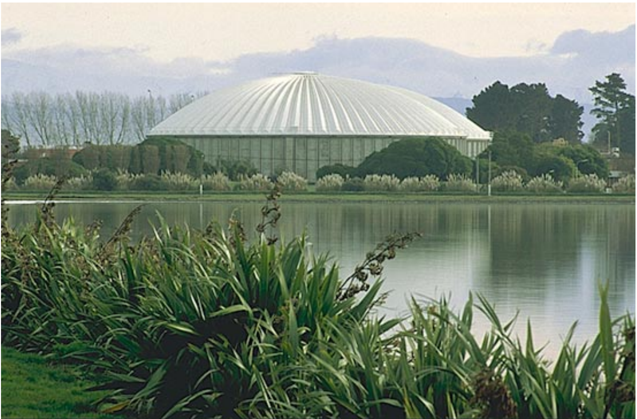
Christchurch Wastewater Treatment Plant showing the covered Trickling Filter and Oxidation Ponds in the foreground.
