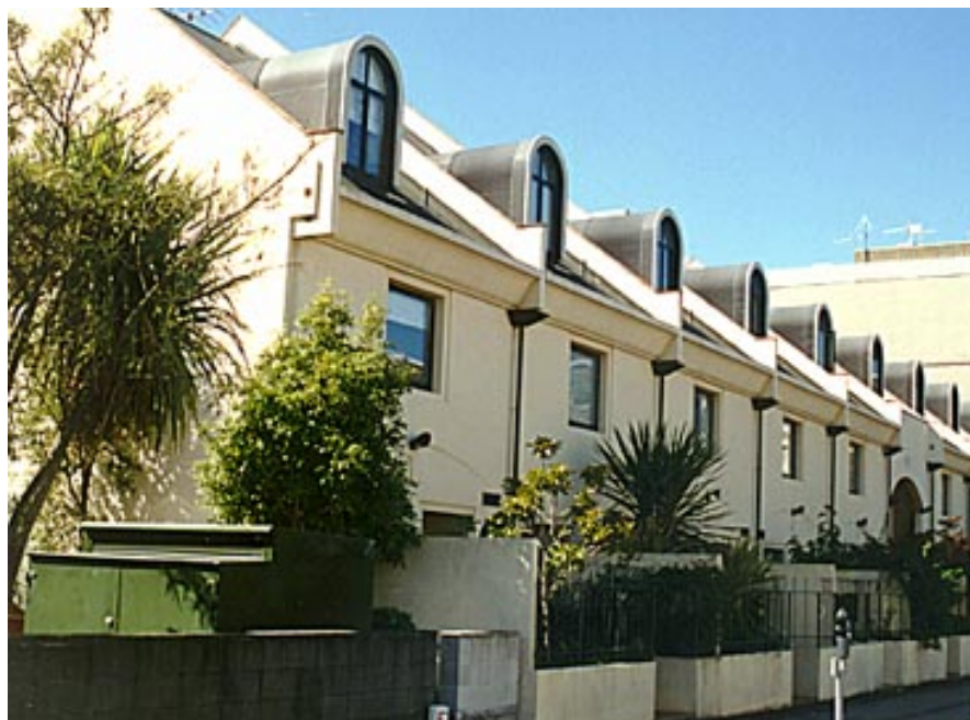
Examples of the redevelopment of Inner City housing.
