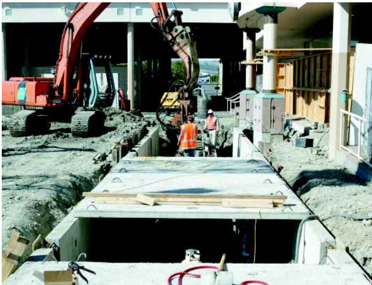
As building work progressed on the Westfield Riccarton mall site, Orion's 66,000 volt cables in the area needed protecting. A concrete tunnel was installed to provide service access to the cables.
