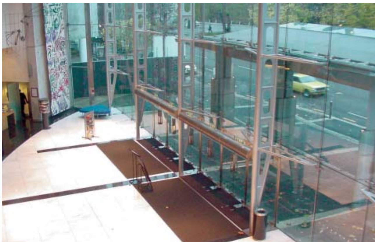
Christchurch Convention Centre Foyer.
