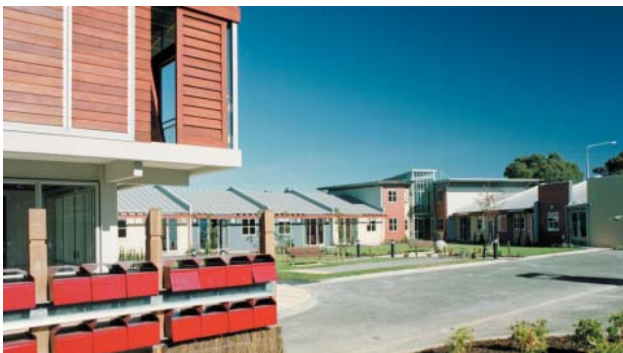
Units forming part of the Council's housing complex in Hornby.
