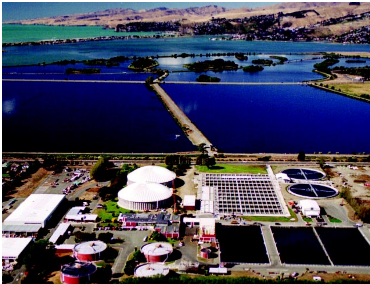
An aerial view of the Bromley Wastewater Treatment Plant
