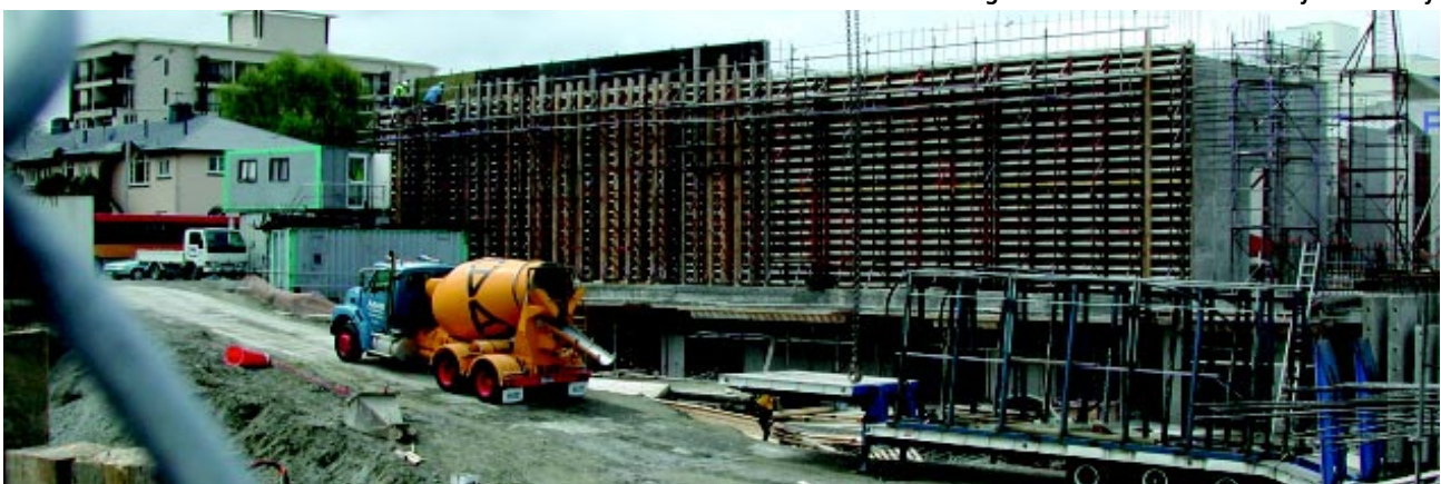
Construction work continuing at the new Christchurch City Art Gallery
