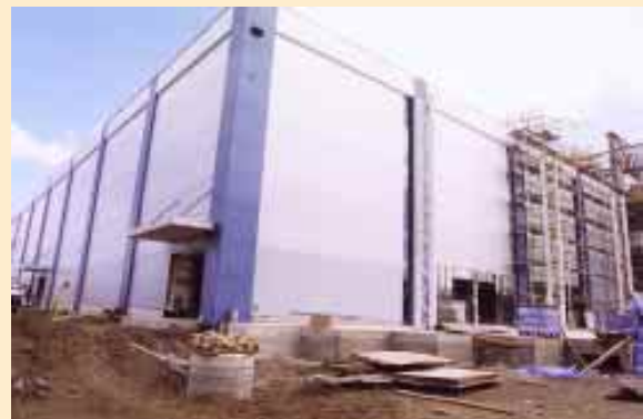
Work is continuing on the redevelopment of the QEII pools
