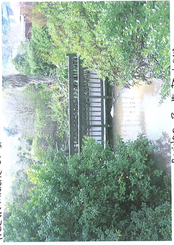
Trees and shrubs overgrown causing turbulence
