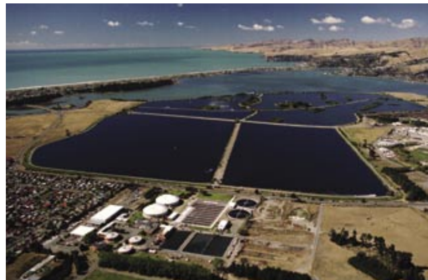
Christchurch Wastewater Treatment Plant
